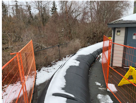
Figure 6-29: Aquadam near Lewis Park (Credit: Ebbwater, 27 Feb 2023).
