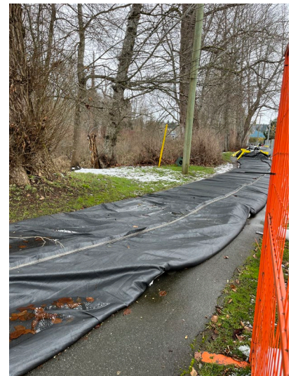
Figure 6-30: Deflated Aquadam (Credit: Ebbwater, 27 Feb 2023).
