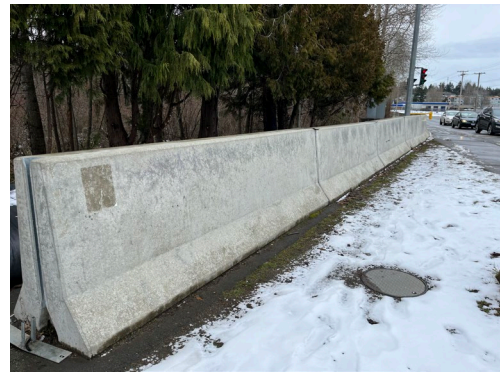
Figure 6-31: Tall Wall along Headquarters Road (Credit: Ebbwater, 27 Feb 2023).
