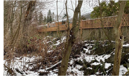
Figure 6-17: Canterbury Lane Dike, with setback concrete wall, riprap toe protection and fencing, with residential complex immediately behind structure. (Credit: Water Street Eng., 27 Feb 2023)
