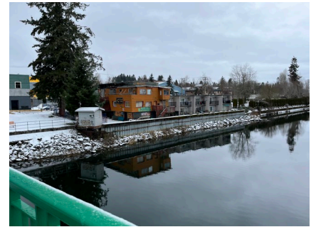
Figure 6-18: Anderton Avenue Dike, view from 5 th Street Bridge. (Credit: Ebbwater, 27 Feb 2023).
