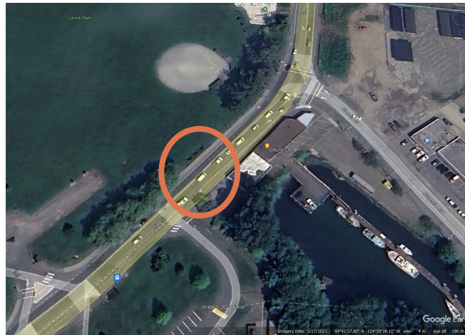
Figure 6-32: Lewis Park Culverts, connecting Lewis Park to Courtenay Slough. (Credit: Google Earth Imagery, 17 May 2023).
