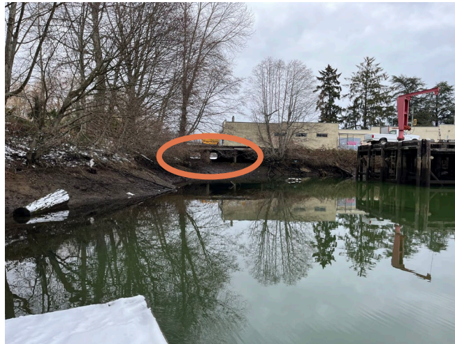
Figure 6-33: View of Lewis Park culverts from the South from Courtenay Slough. (Credit: Ebbwater, 27 Feb 2023).
